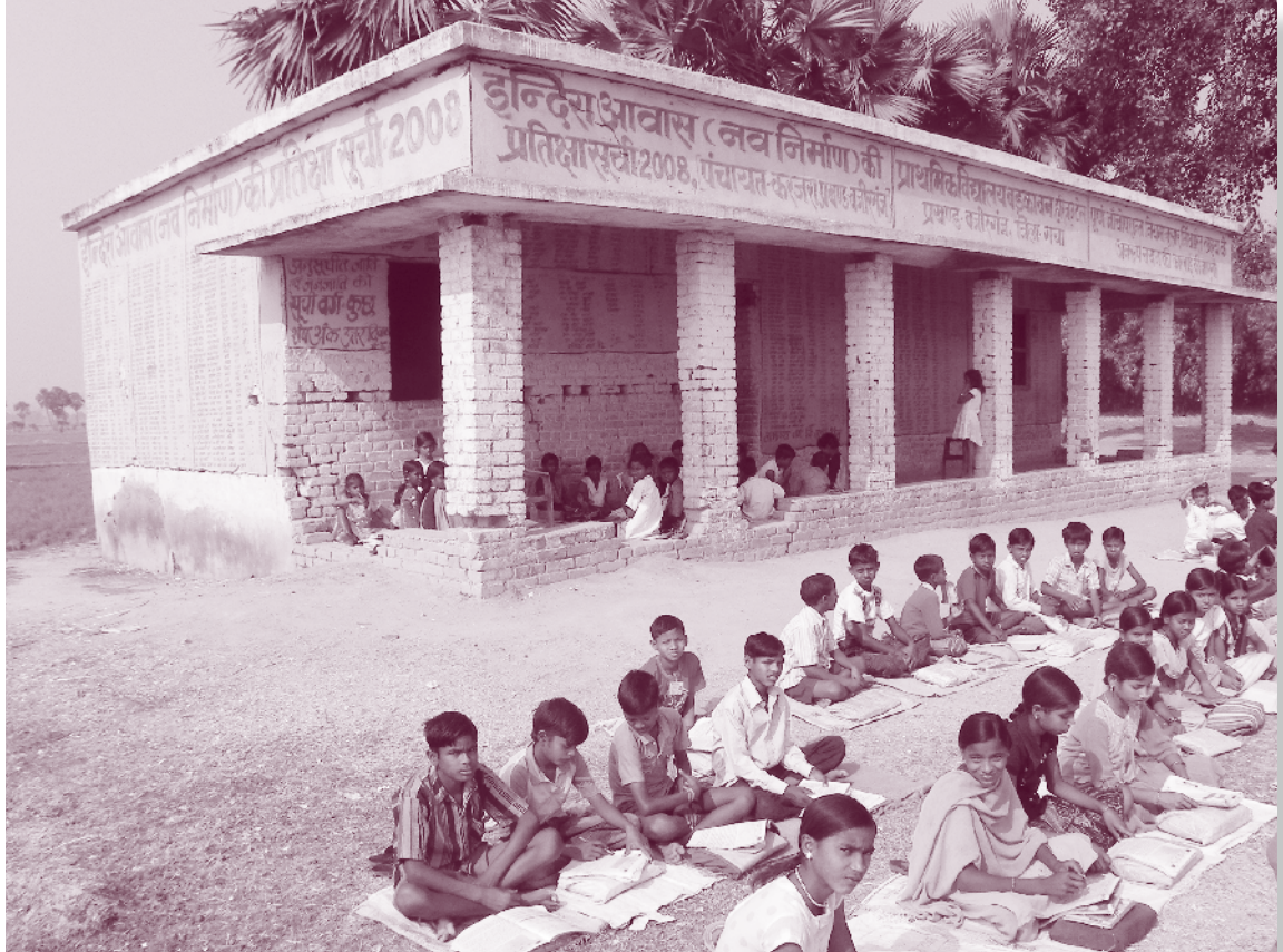
Inadequate Number of Classrooms for children in Badka Bandh
