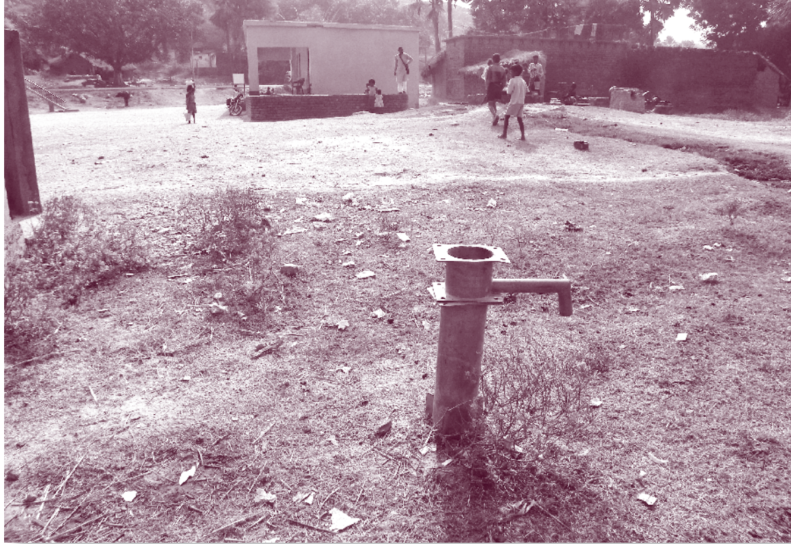
Broken handpump in school at Majhauri
